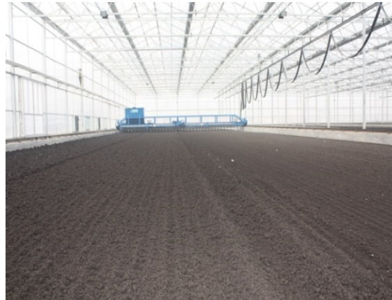
Solar sludge drying
